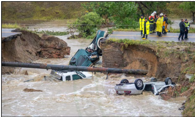
Figure 8 Illustration of streambank and channel erosion
