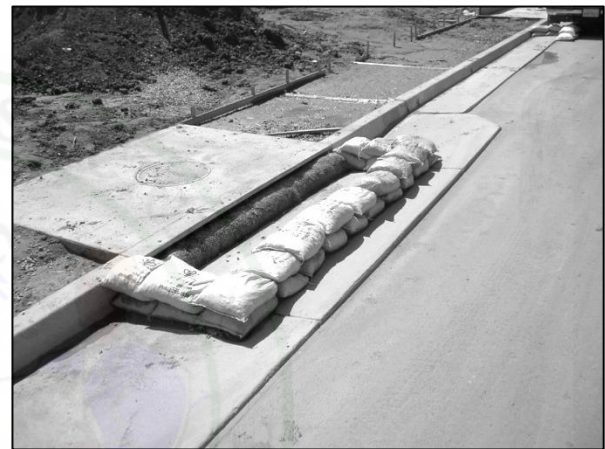
Figure 2 BMP installed on the construction site
