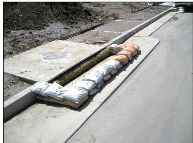
**Figure 1** Detail from the ESC drawing
