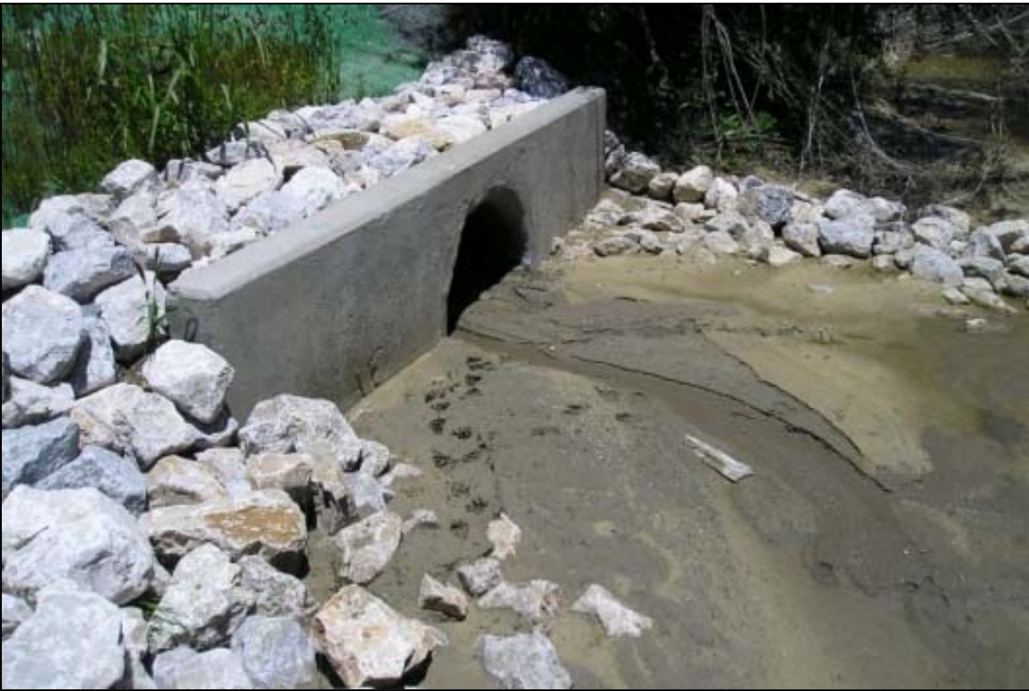
LOCATION J (LOOKING SOUTHWEST, STANDING IN THE PRE-SEDIMENTATION BASIN)
