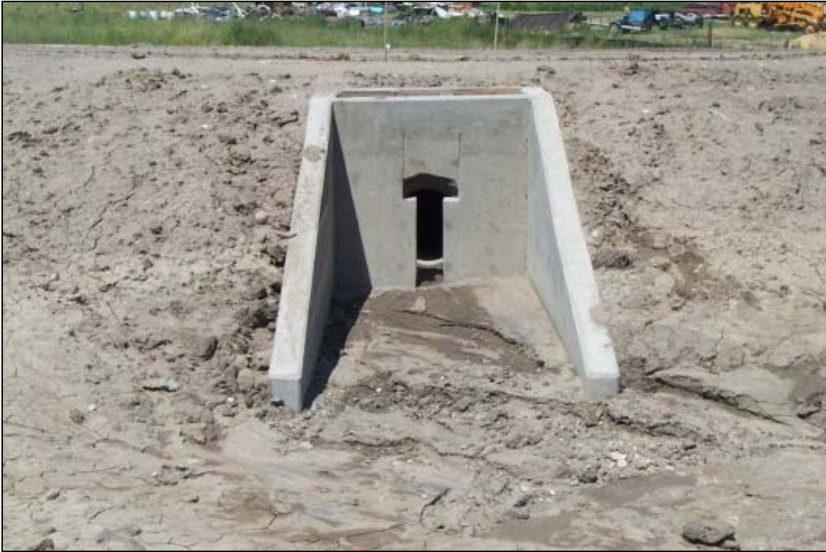
LOCATION K (LOOKING NORTH)
