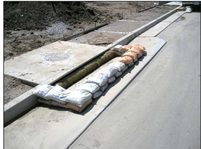
Figure 2 BMP installed on the construction site
