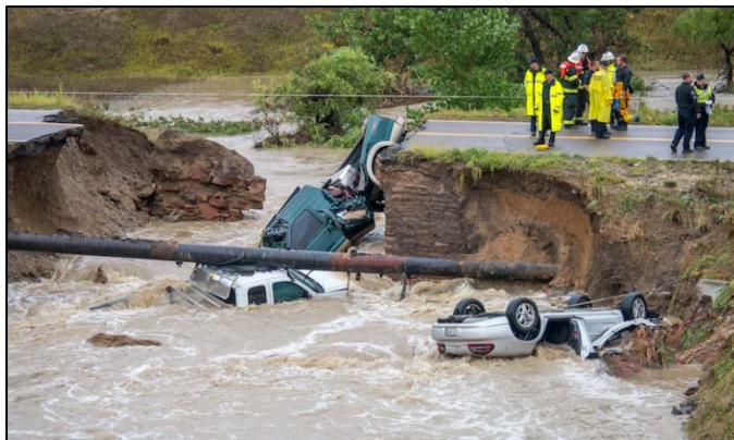
Figure 8 Illustration of streambank and channel erosion
