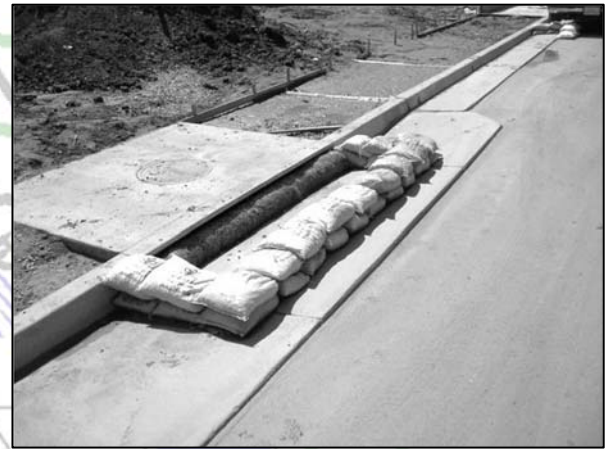
Figure 2 BMP installed on the construction site
