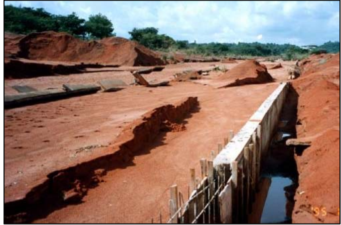
Figure 7 Illustration of a gully on a construction site
