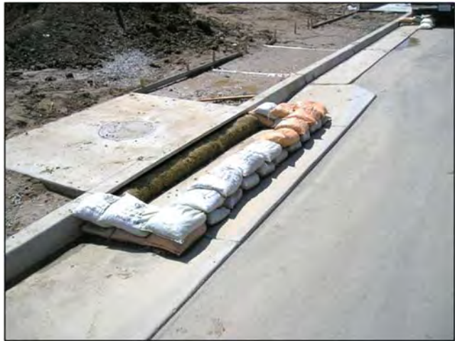
Figure 2 BMP installed on the construction site
